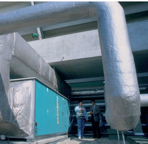
Circulating pumps for building management
